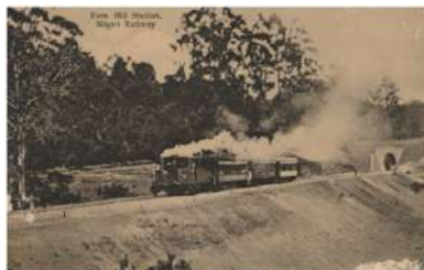
Figure 6: NMR at Fernhill Station
