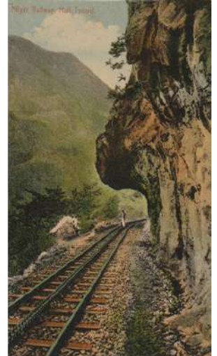
Figure 10: Rack bars between the track rails of NMR
